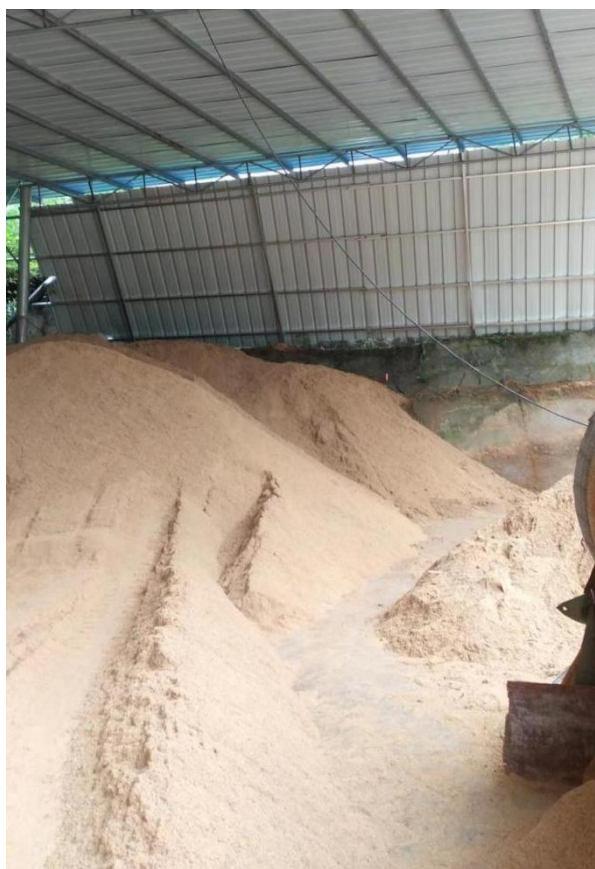
半封闭原料棚
